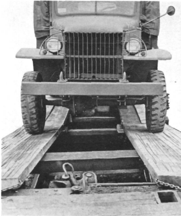
Fig. 2—A 2½-ton takes the high road. The runway of the ramp is built of 3×12's.
